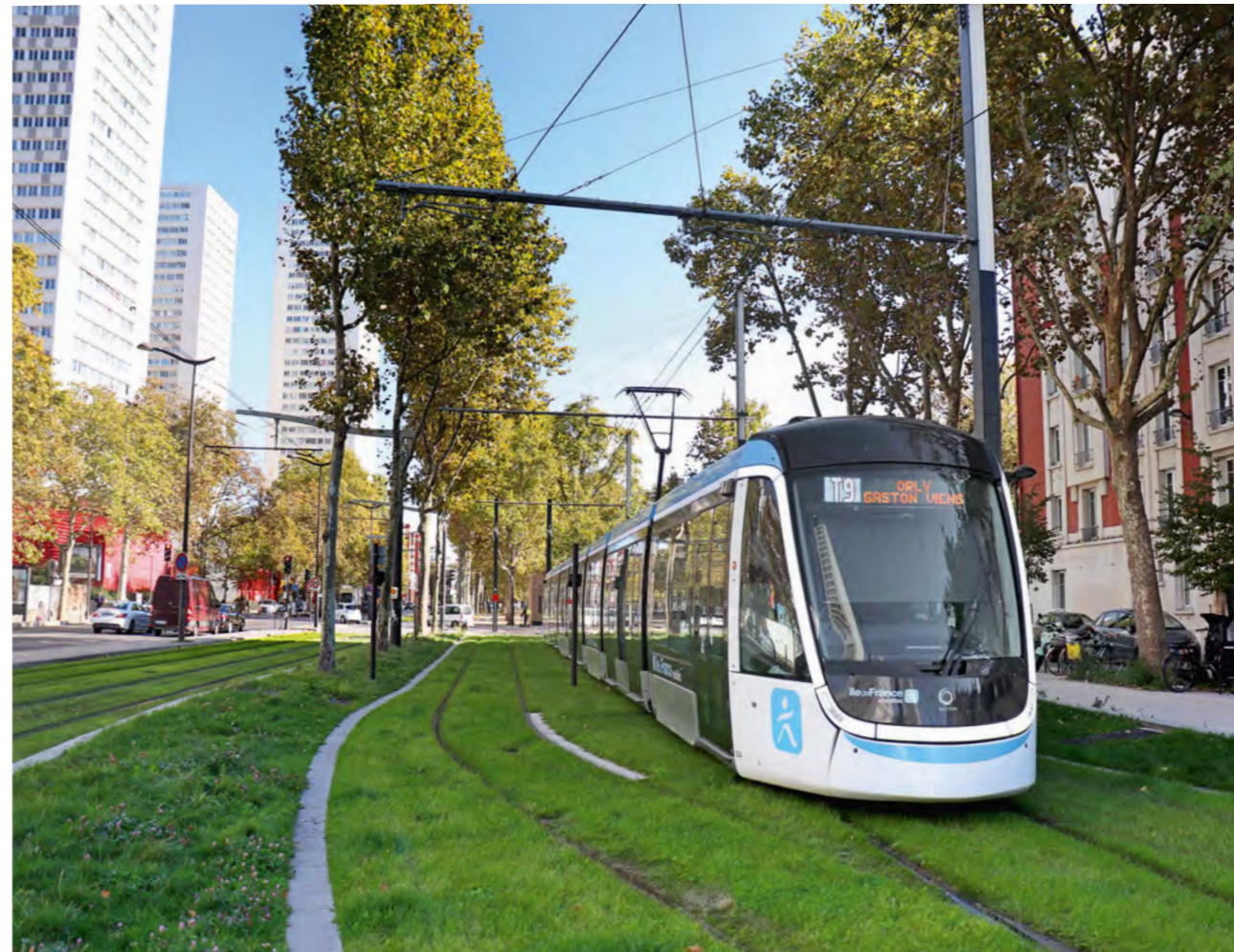
← Soft green track beds along the new T9 tram line in Paris.
