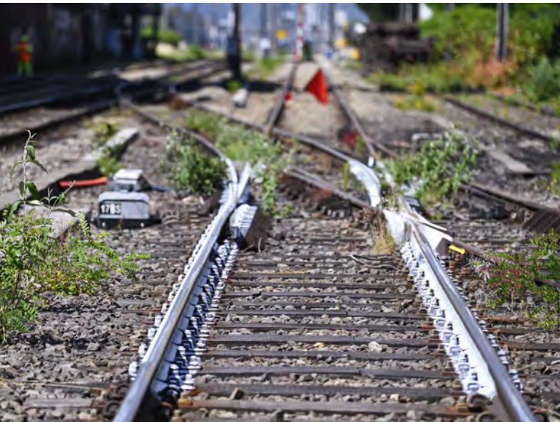
← Rails painted white during the 2022 heatwave, Liège, Belgium.
