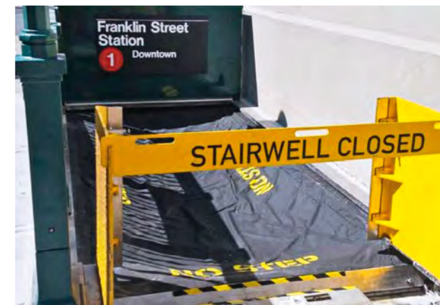
← Flexible, water resistant flood barriers on an entrance to the New York subway.
